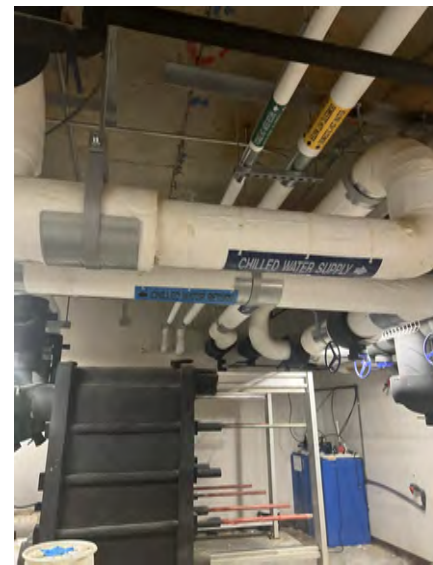
CHILLED WATER SUPPLY PIPES (BASEMENT)
