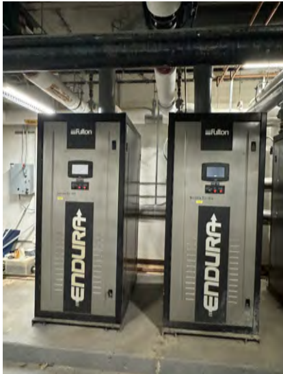
BOILER FOR HEATED WATER SUPPLY
