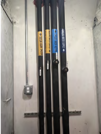
HEATED AND CHILLED WATER SUPPLY PIPES
