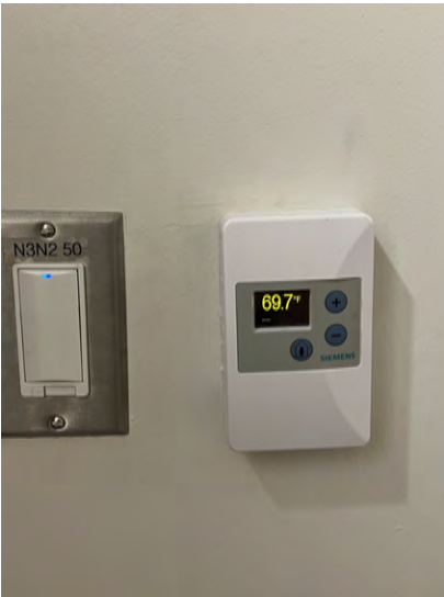
INDIVIDUAL ROOM TEMP. CONTROL THERMOSTAT
