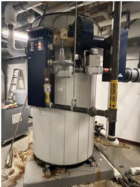
WATER HEATER STORAGE TANK WITH NATURAL GAS LINE
