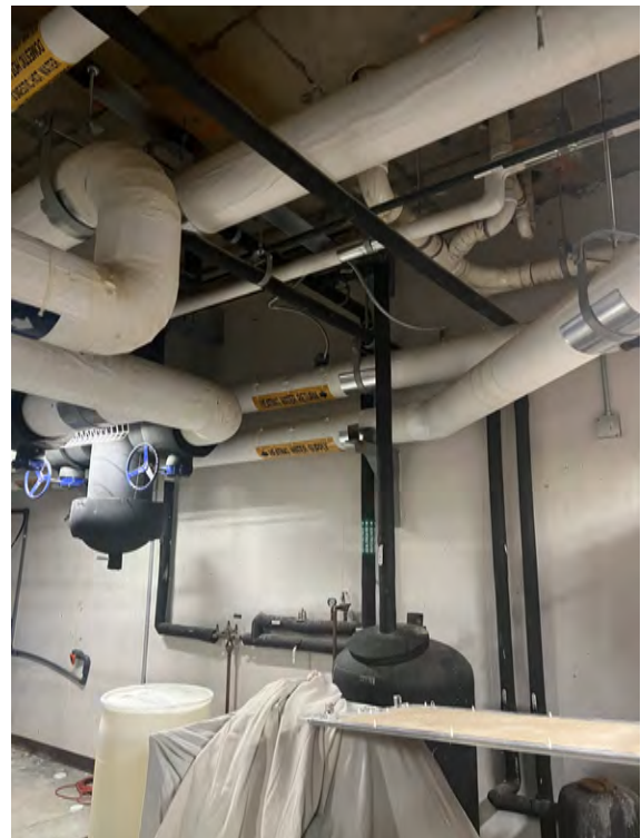
DOMESTIC HOT WATER PIPES
