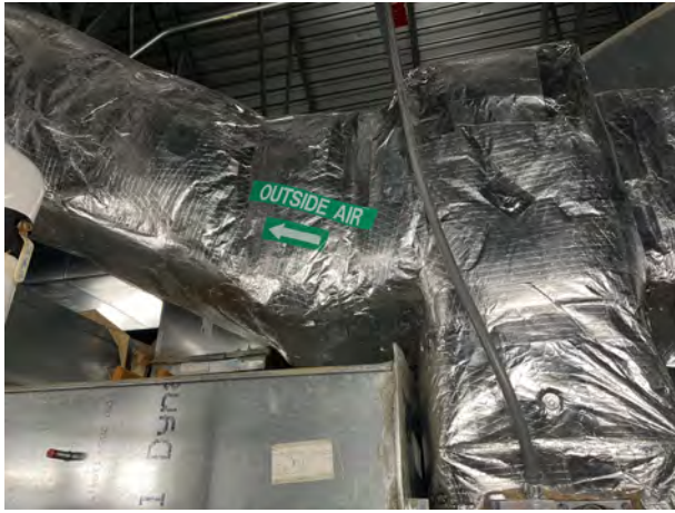
OUTSIDE AIR SUPPLY DUCT WORK
